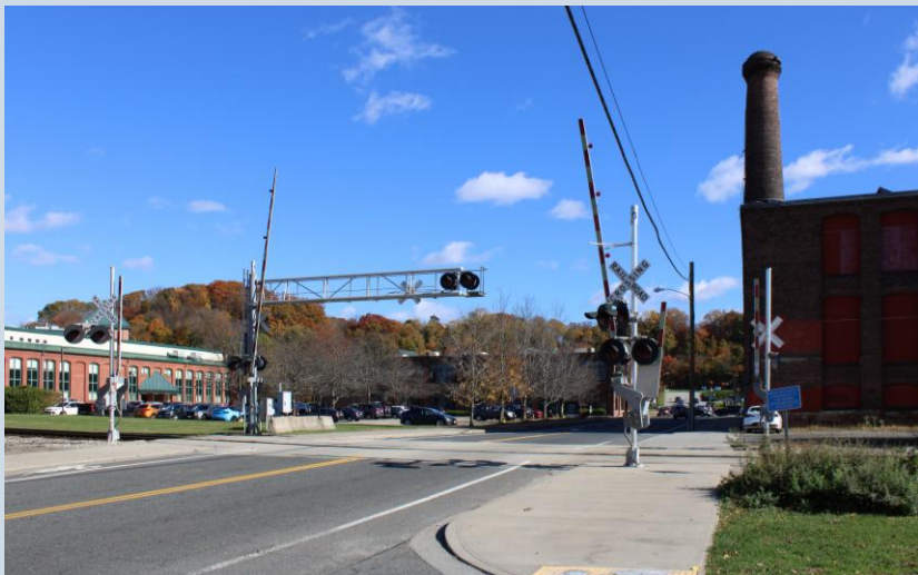
The railroad crossing at Wason Avenue is one of only two roadway connections between the Brightwood neighborhood and the rest of the city
