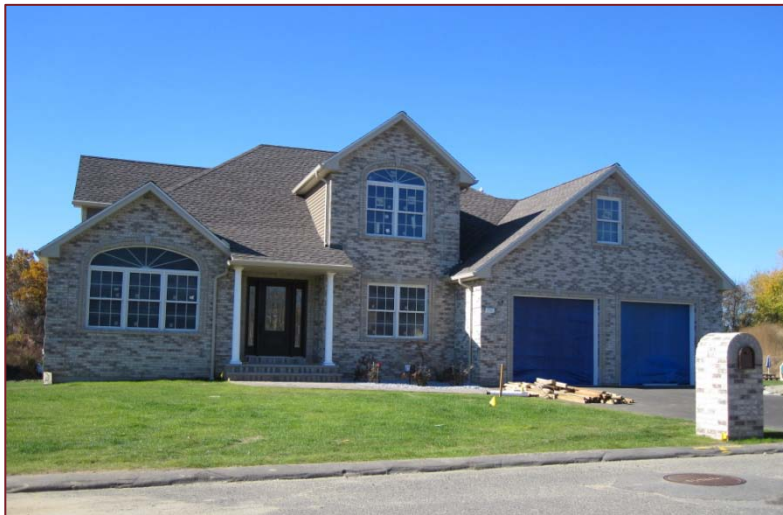
Image 12: A single family home under construction in Chicopee. Source: City of Chicopee, 2013
