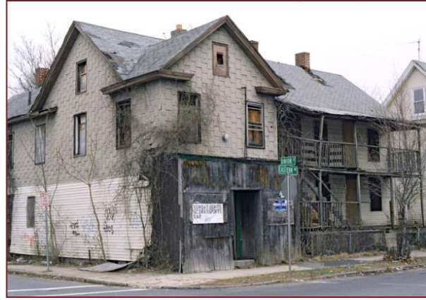
Image 6: a vacant, deteriorating house in the Old Hill in Springfield, at Eastern Street and Union Street. Source: HAPHousing, Inc.
