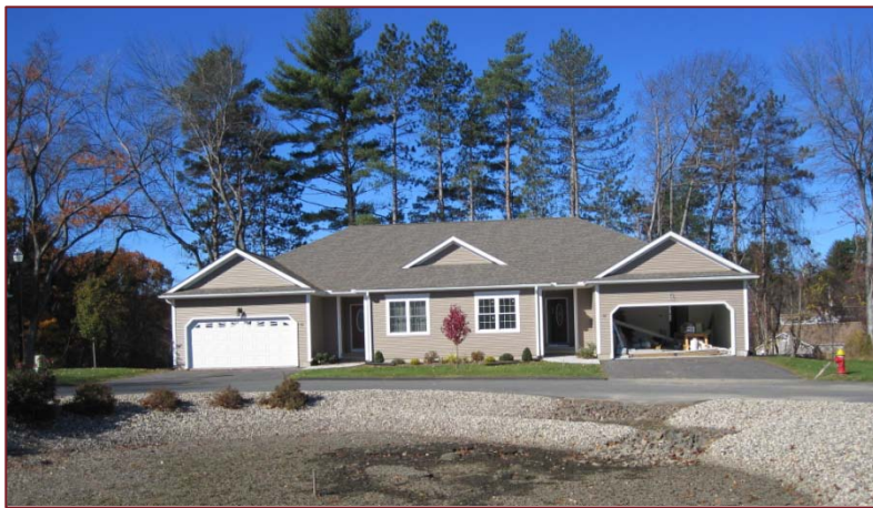
Image 11: Two family condos under construction in Chicopee. Source: City of Chicopee, 2013
