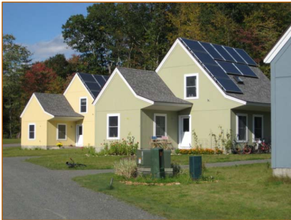
Image 27: Laurel Road Condominiums in Haydenville is an example of a “higher” density residential development in a rural community. Source: PVPC
